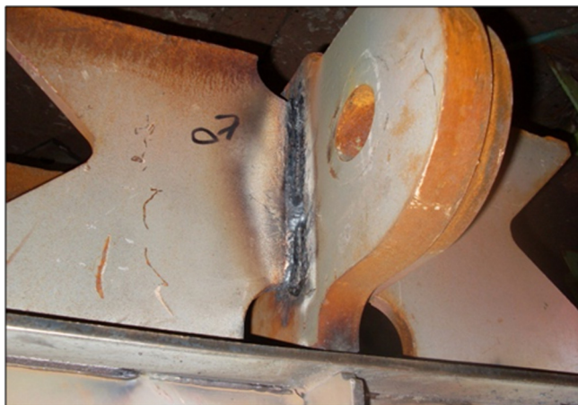
(b) Lug hole and double plate
