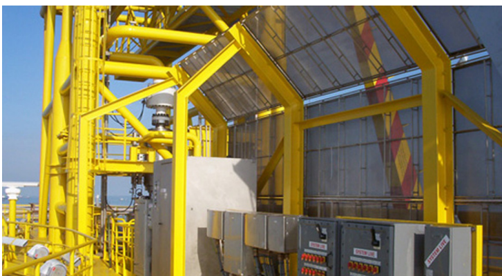
Fig. 1 Applications of radiant heat shield products (Source: www.heatshielding.com; www.esterline.com)
