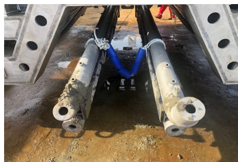
Damaged jetting arm
