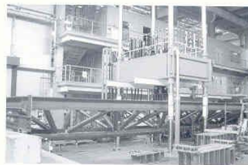
▲[사진 2] Tubular Joint
